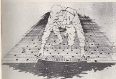
**Ceramic Wall Panels with flexible grouting.** One-inch modular unglazed mosaic ceramic tiles chemically coupled in a flexible urethane matrix, formed in a two-by-two-inch panel that installs with organic adhesive using resilient tile techniques. "TiRamic" manufactured by Monsanto.
