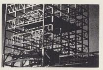
Staggered Steel Truss System. Steel framing system uses series of story-high trusses spanning between perimeter column lines. Trusses are placed in a staggered pattern so that the floor system is supported by the bottom flange of one truss and the top flange of the next truss.
