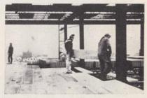
Metal Edge Gypsum Plank Floor System. Consists of T & G plank 2 inches thick by 15 inches wide by 10 feet long, installed as a welded-together deck over 24-inch o.c. bar joists. Gypsum mastic topping is provided as a floor leveling material and %" gypsum boards on furring channels are installed at the bottom of joists for a two-hour fire rating. Manufactured by U.S. Gypsum Company.
