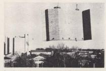
Single Wythe Masonry Wall System, Uses a latex additive to Types I or III Portland Cement high bond mortar, When mixed with "A" marble dust or Etu Dolomitic limestone, it produces a high bond mortar with both high compressive strength and high tensile or flexural strength—when considering resistance to lateral or beam loadings. "Sarabond" manufactured by Dow Chemical Company.
