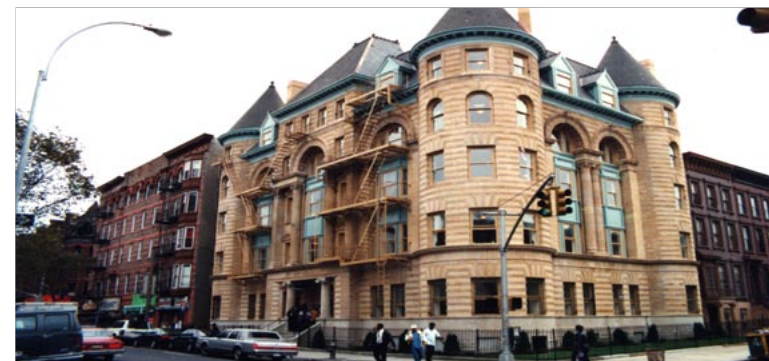
In 1995, after redevelopment In 1998, after redevelopment In 1999, after redevelopment
